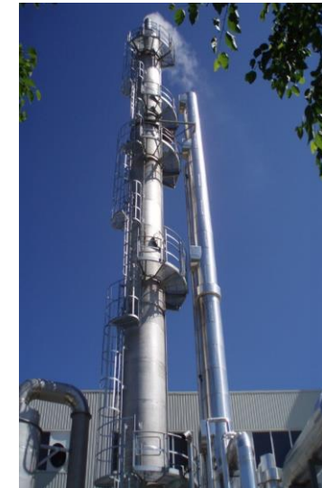
Amine absorption system
